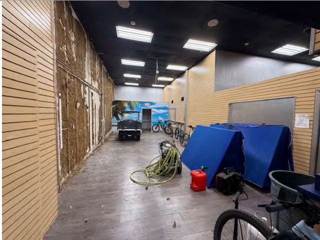
Marine Stadium Marina – Retail Building
