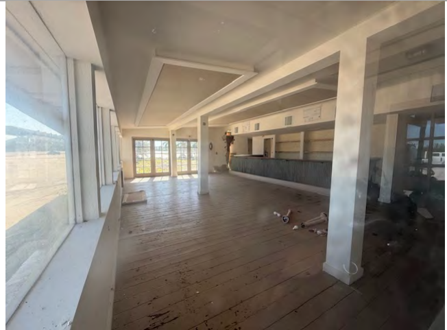
Marine Stadium Marina – Retail Building
