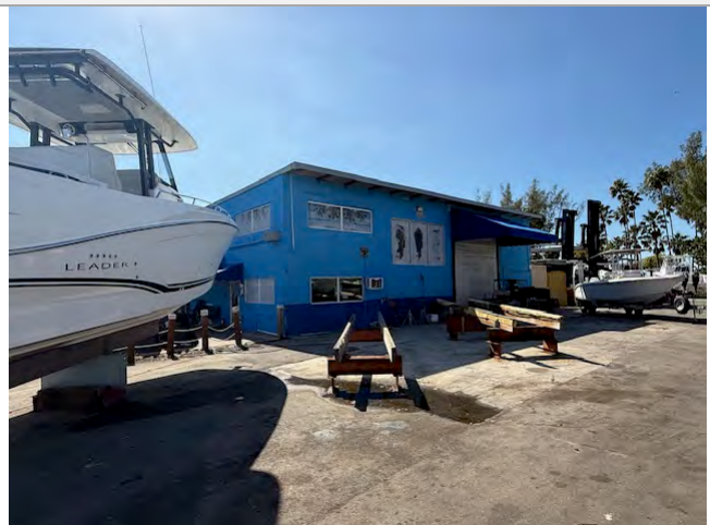
Marine Stadium Marina – Retail Building
